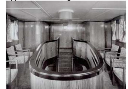
Upper Saloon looking aft.
