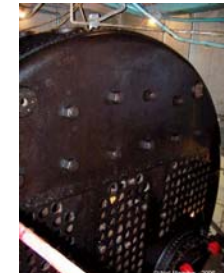
Another view showing the conservation of the boiler shell.
